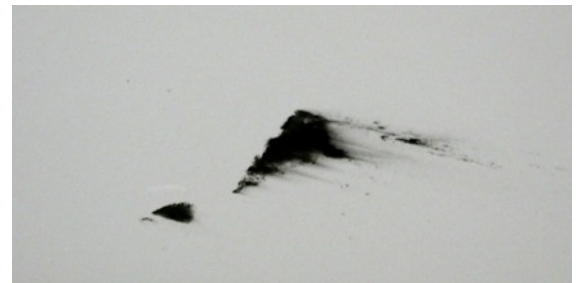
Ricochet mark on kitchen ceiling
